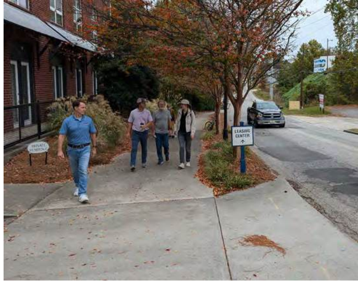
The sidewalk in front of 200 Collier Road apartments is one of the highest quality segments along the corridor. It is wide enough for people to walk side-by-side, has a planted buffer, and is set back far enough to allow for level crossings at driveways.
