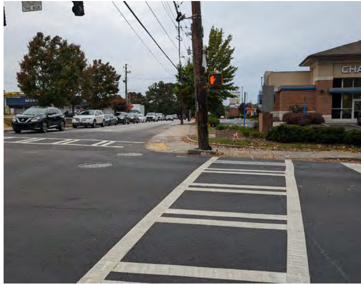
At Howell Mill Road, there are high-visibility crosswalks at all four legs of the intersection with pedestrian signal heads.
