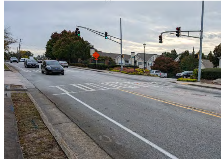
The signalized intersection with crosswalks shown is placed in front of Willowest Apartments on Collier Road so that pedestrians can cross the street safely from their homes and drivers can turn into traffic.
