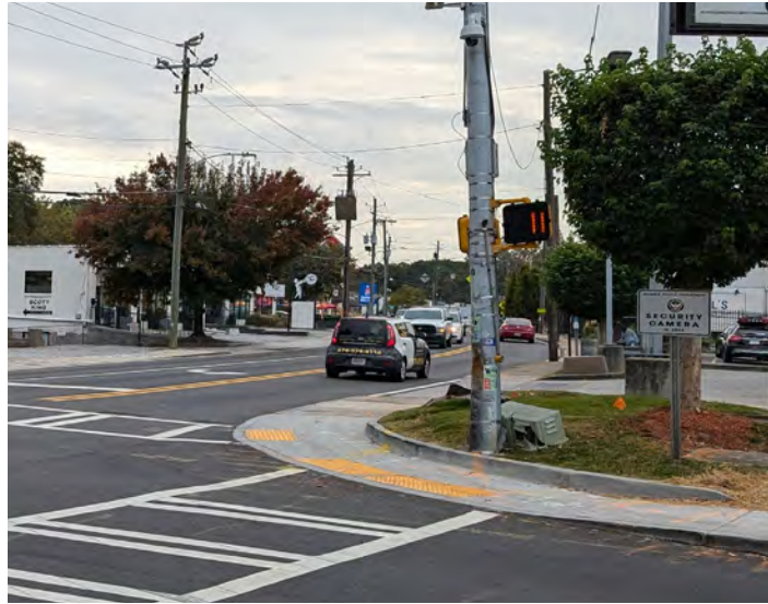
At Howell Mill Road, tire marks on the curb behind the sidewalk are evidence that large trucks are using the full pedestrian waiting area / sidewalk to make the turn from Collier Road to Howell Mill Road.
