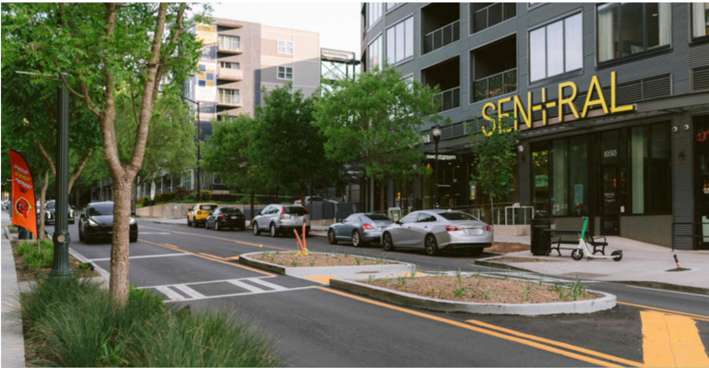
Similar streetscape along nearby Howell Mill Road with: a wide sidewalk, a landscape buffer with pedestrian lighting, a center left turn lane with a pedestrian refuge island awaiting an RRFB and landscaping
